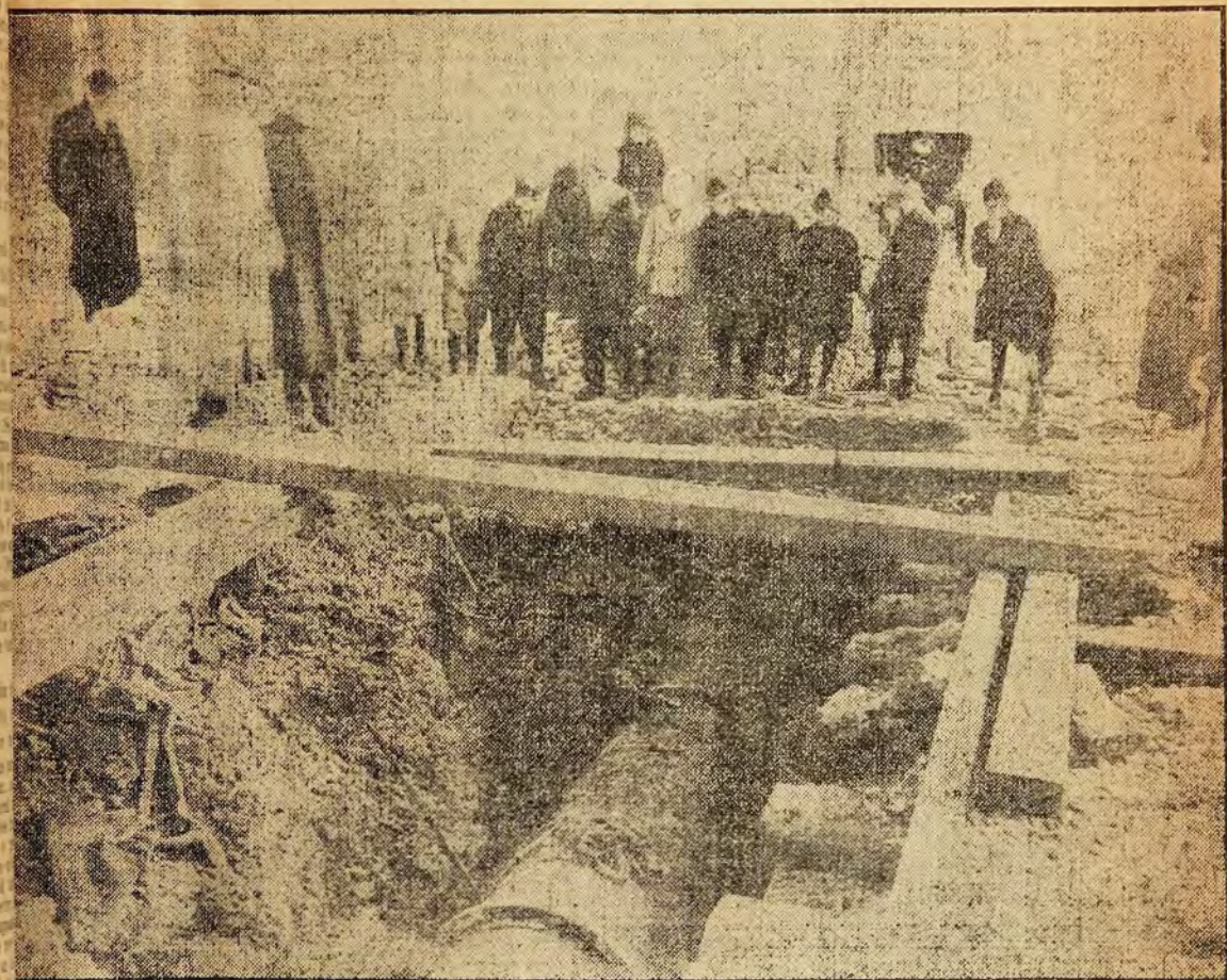
SECTION OF PIPE SHOWING THE BREAK.
